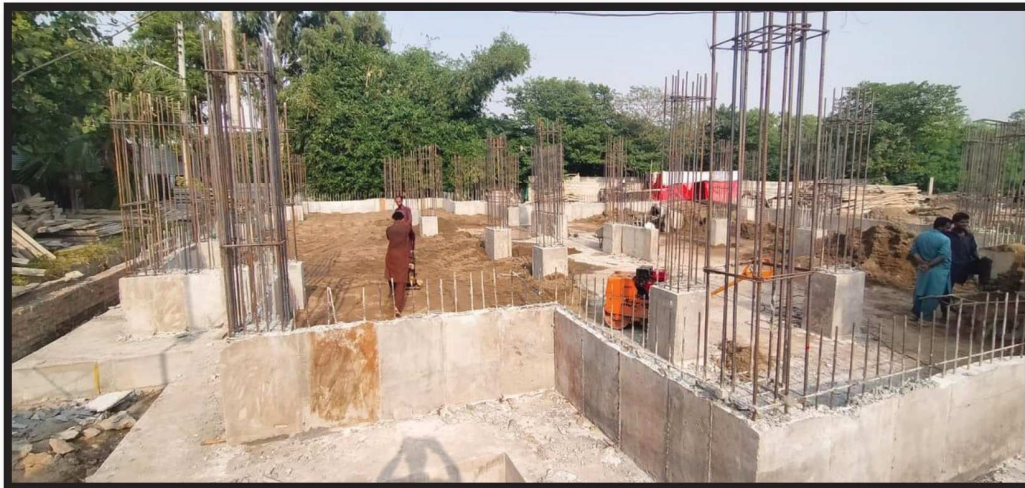
COLUMN,R.C.C WALL.SHEAR WALL UP TO PLINTH LEVEL WORK COMPLETED OF STAFF ACCOMMODATION
